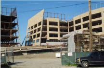
When the office space called 409 and 499 Illinois was planned for San Francisco's Mission Bay area, it faced considerable waterproofing challenges. Two six-story towers were to be constructed over a three-levelsubterranean parking garage that was adjacent to a filled-in turn-of-the-century shipping channel that provided a water infiltration conduit from the bay to the garage.
